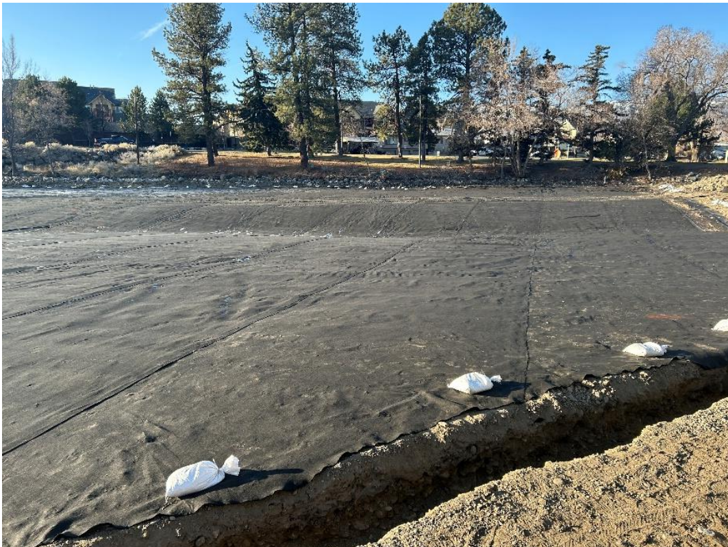
New Pond liner installed
