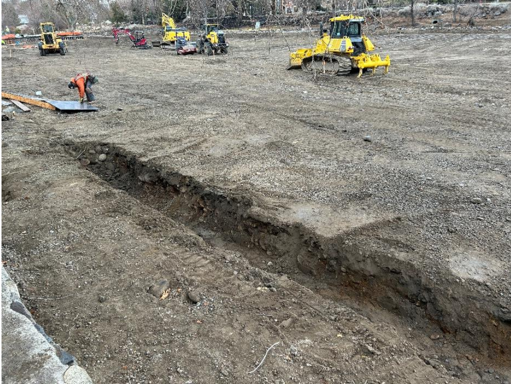
Drained Pond and crews are preparing for the new liner
